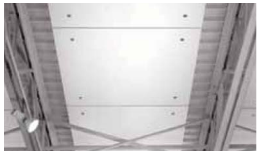
OPTRA Capz, installed 70mm from a metal deck.
