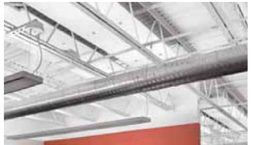
OPTRA Capz, installed 165mm from a metal deck.
