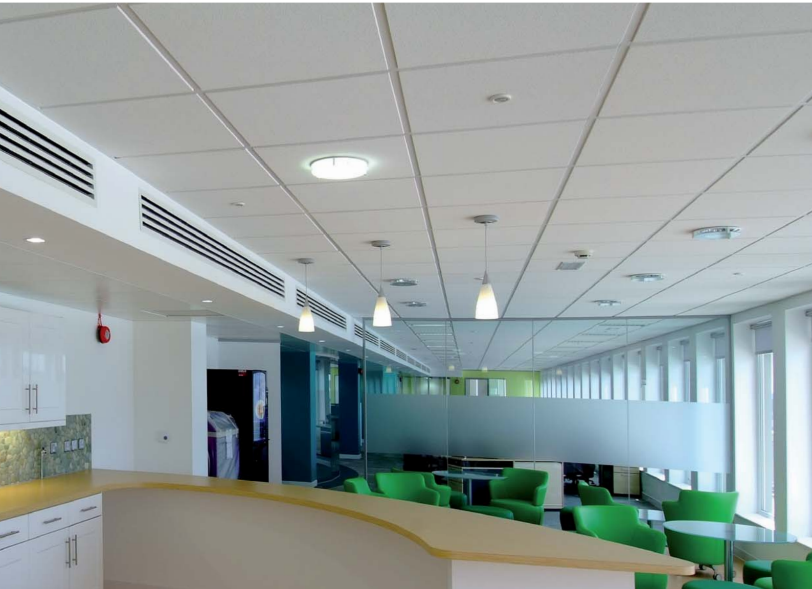
DUNE Angled Tegular with Peakform Prelude XL 24mm Exposed Tee Grid
