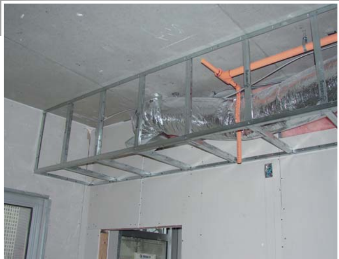
Right: QuikStix Bulkhead Installation in progress
