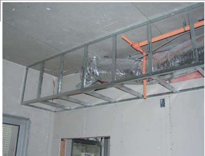
Right: QuikStix Bulkhead Installation in progress
