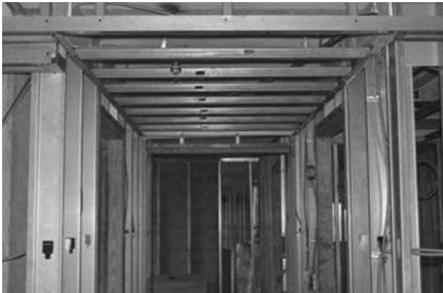
Corridor framing using traditional steel studs
