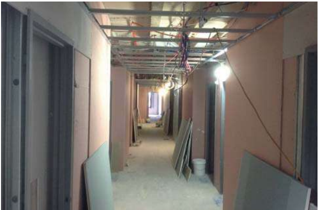
ShortSpan Framing and Locking Angle Moulding make drywall framing faster and easier
